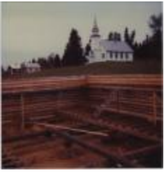
Old Fort Community Hall (2018.2.30.05)
