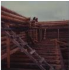
Old Fort Community Hall (2018.2.30.04)
