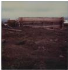
Old Fort Community Hall (2018.2.30.03)
