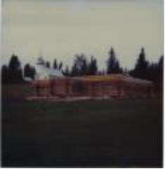
Old Fort Community Hall (2018.2.30.06)
